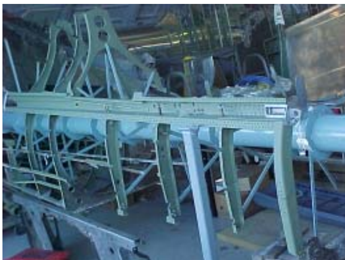
Top longerons & front frames rebuilt
