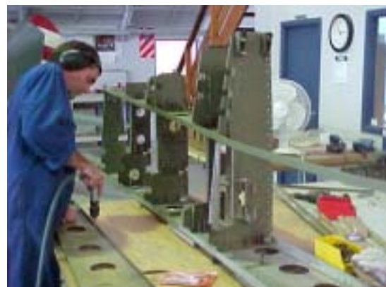
The components of the structure from Spar 3 to 5 are being rebuilt systematically
