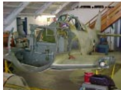
17-Systems & plumbing fitted
